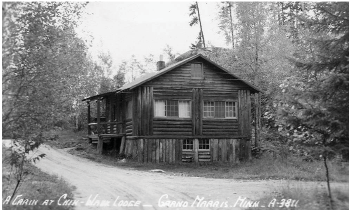
Figure 2- 66: Old Lodge (#12 Cabin), early view with log foundation. This was the first lodge at the property and it faced the road, rather than the lake shore. (source: C-W 26, This post card is from Norbert Mayer.)
