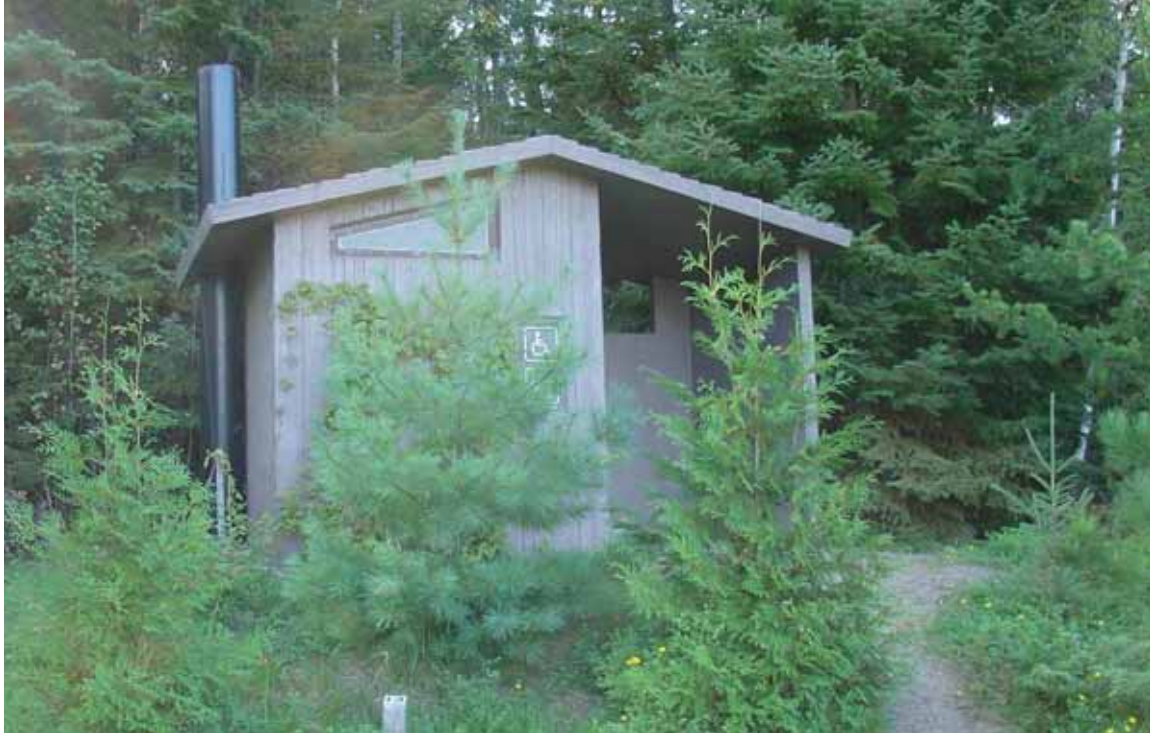
Figure 4- 33: Outhouse at Chik-Wauk, August 2012 (source: OEA)
