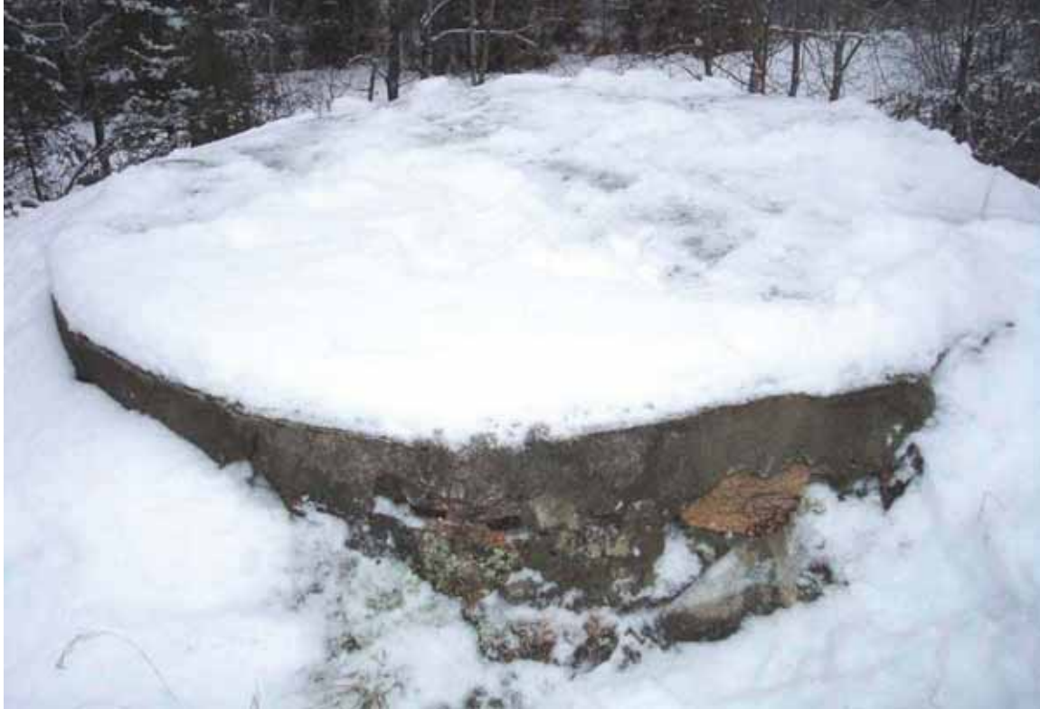
Figure 4- 39: Stone and cement circular foundation of former water tank, December 2012 (QEA)
