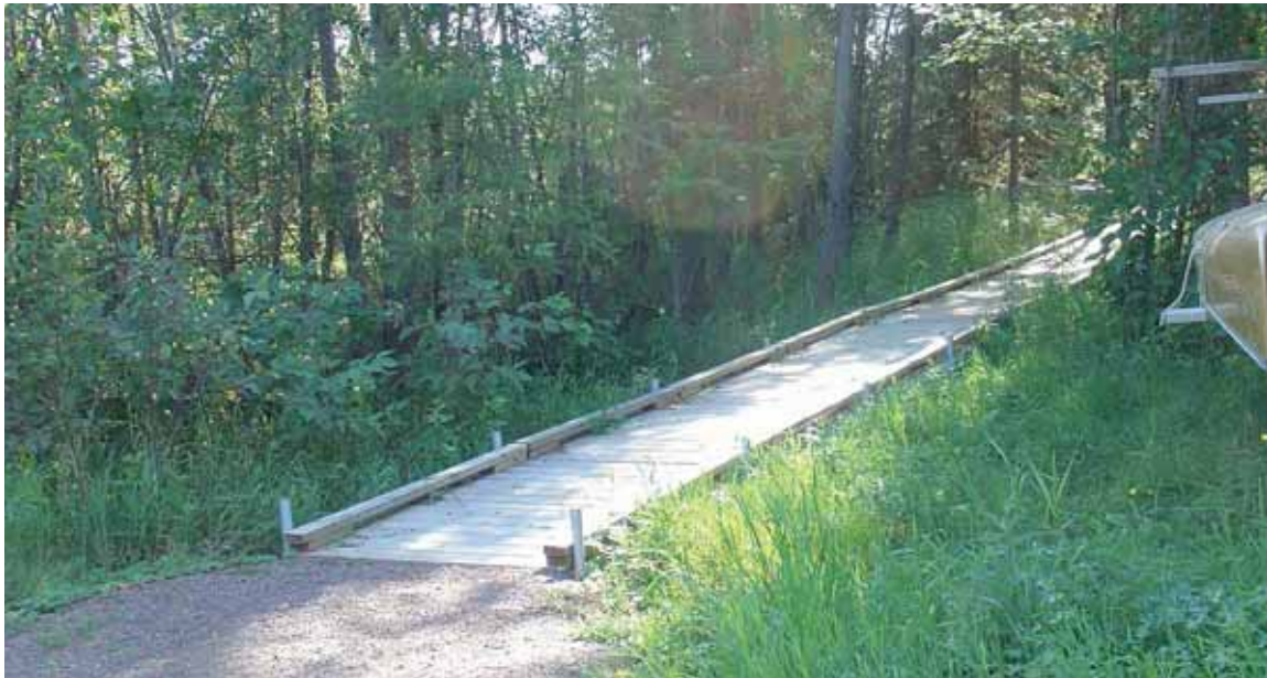
Figure 4- 41: Boardwalk near relocated canoe trip outfitting building, August 2012 (source: QEA)
