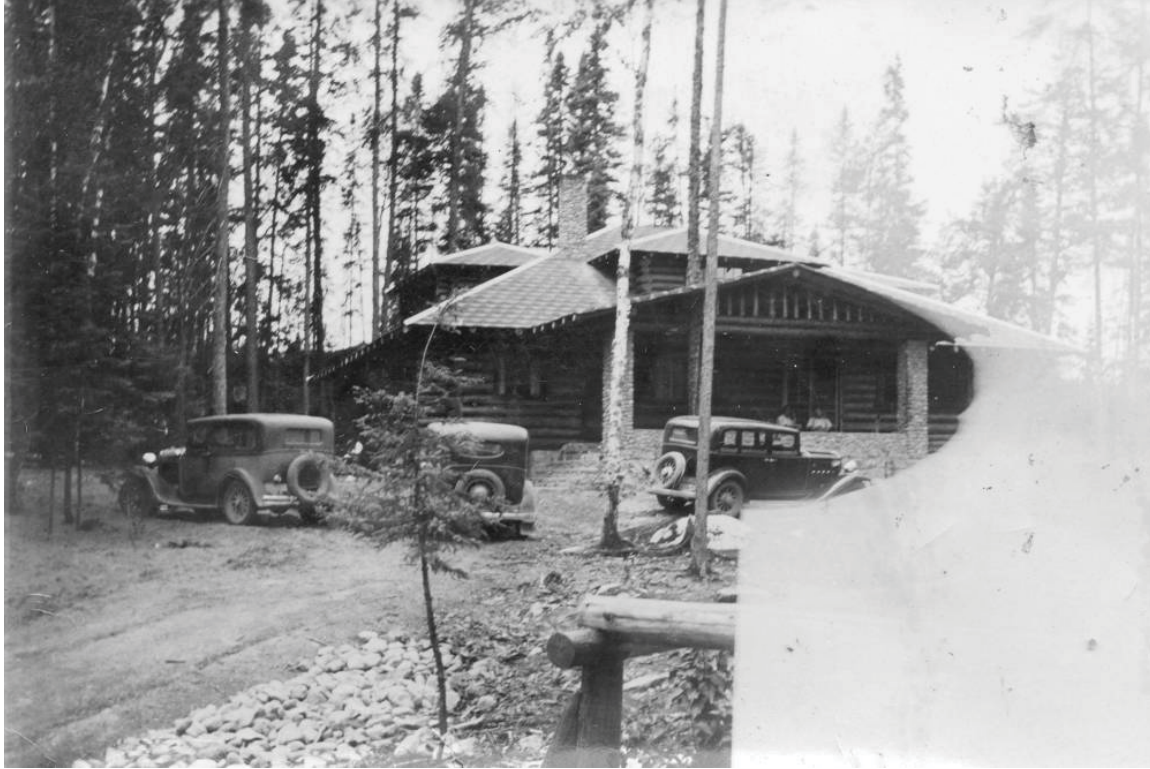
Figure 2- 2: Second Chik-Wauk Lodge (first building in this location), constructed of logs with stone porch, ca. 1932 or 1933. (source: C-W 198)
