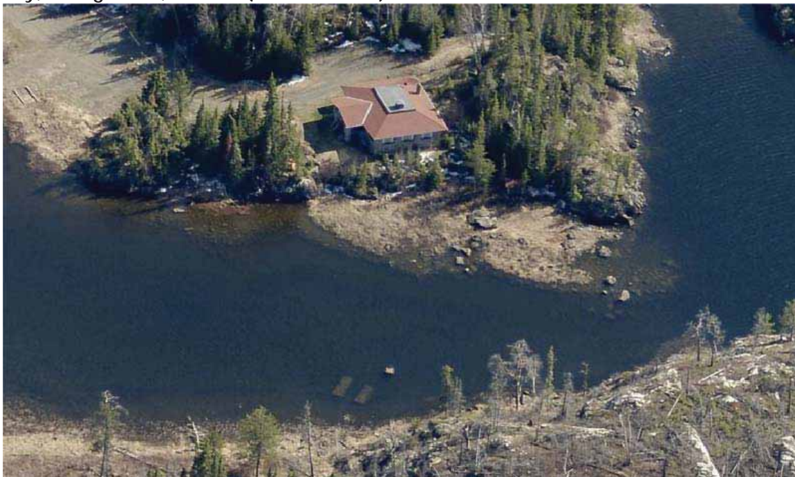
Figure 4- 21: EV#7, Existing oblique aerial View of Chik-Wauk lodge and surrounding area from across the bay, facing south, 2013 (source: Bing Maps)
