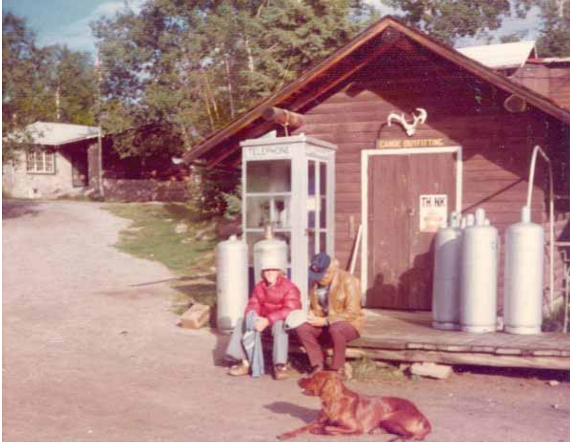
Figure 2- 41: Canoe Trip Outfitting Building, 1974 (source: C-W 188)
