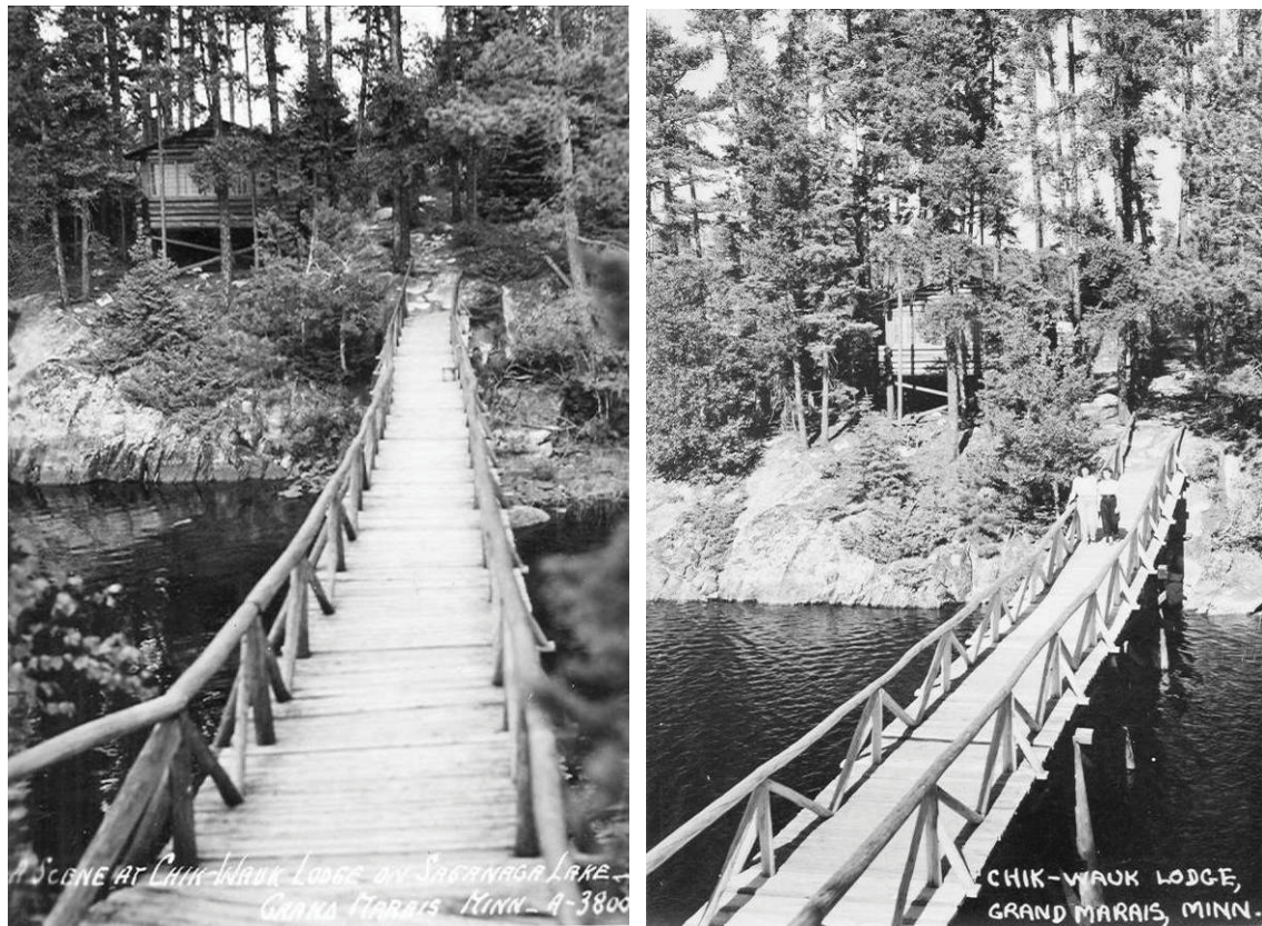
Figure 2- 58: Footbridge at Chik-Wauk with Judge's Cabin (#2 Cabin) on left. (source: left C-W 21, right C-W 45 & same as C-W 54)
