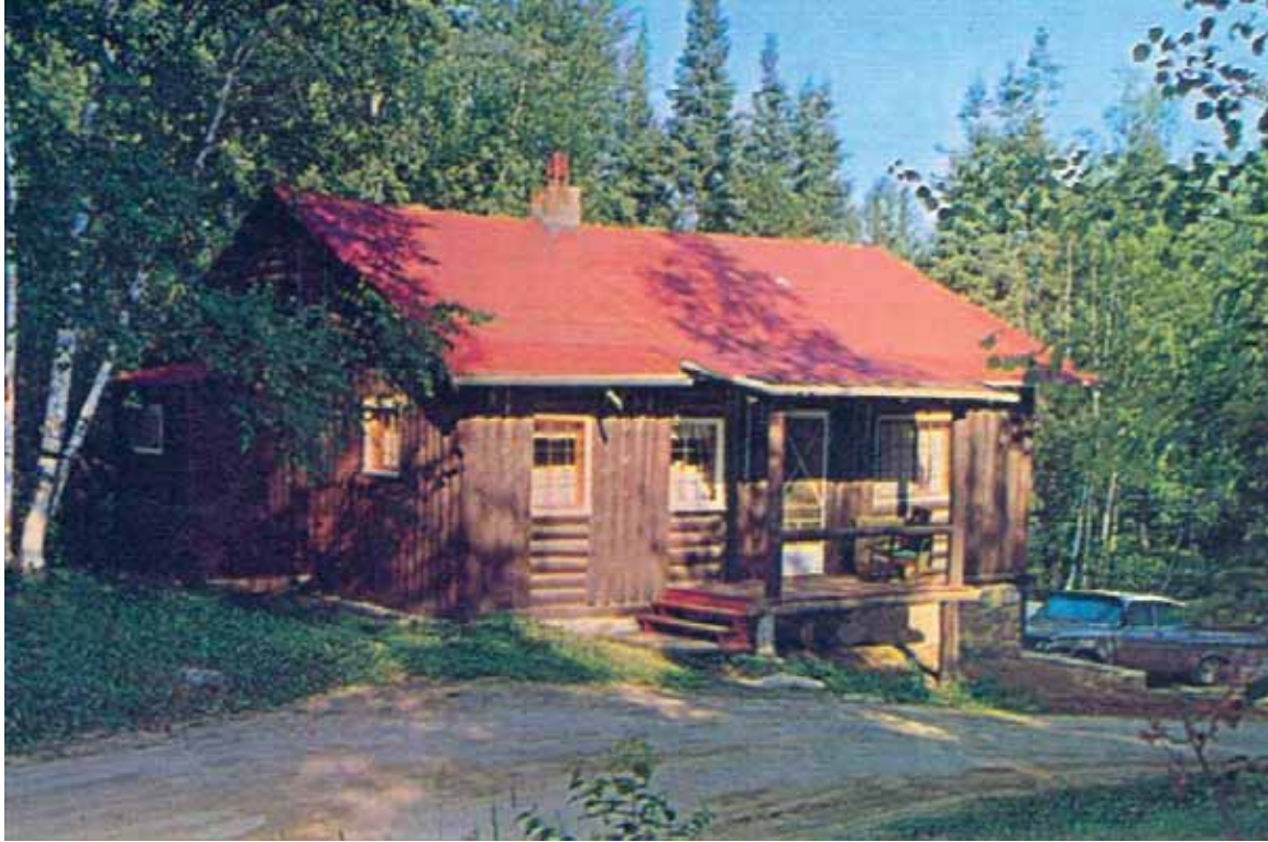
Figure 2- 68: Old Lodge (#12 Cabin), later view with stone foundation. (source: C-W 46, picture is from Sharon Eliassen)
