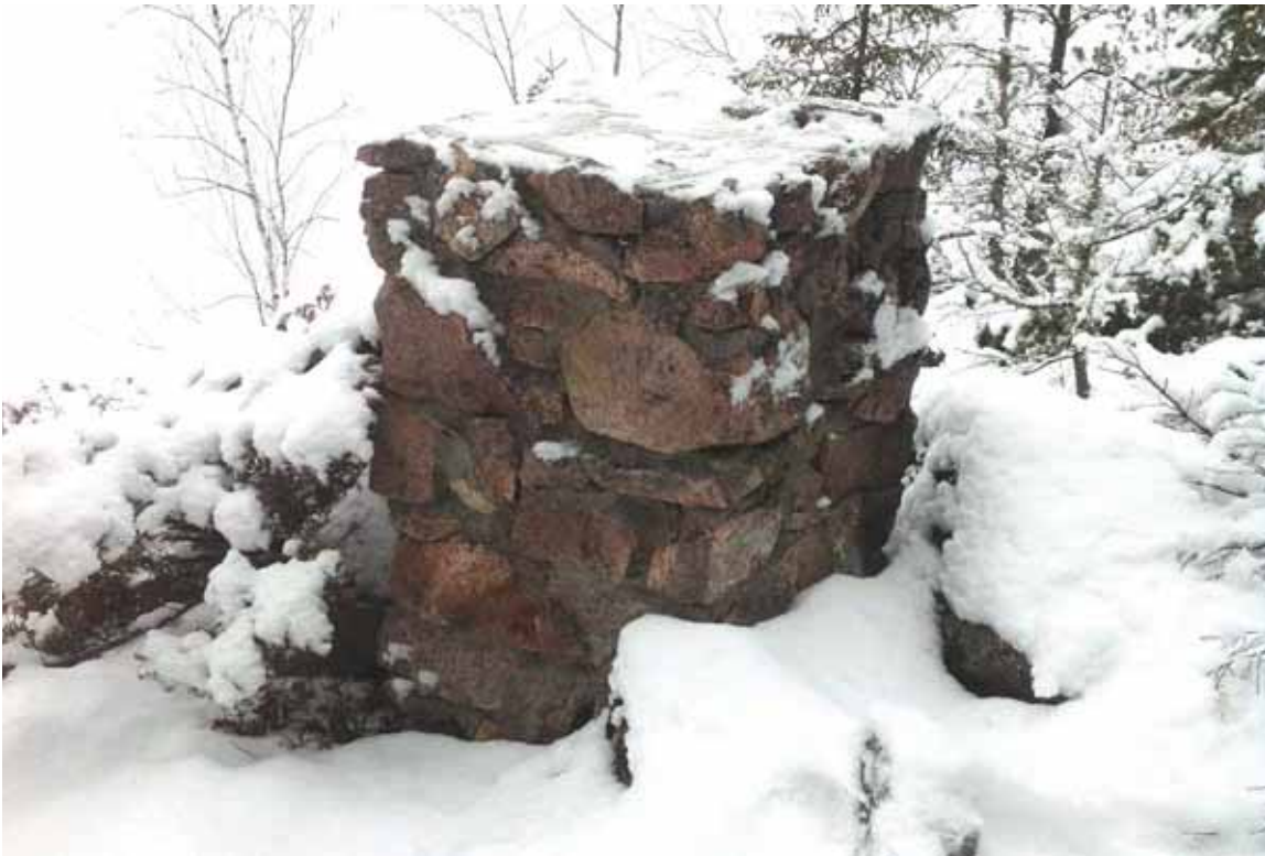
Figure 4- 36: Mortared stone foundation pillar at former Carey Cabin (#1 Cabin ), December 2012 (QEA)
