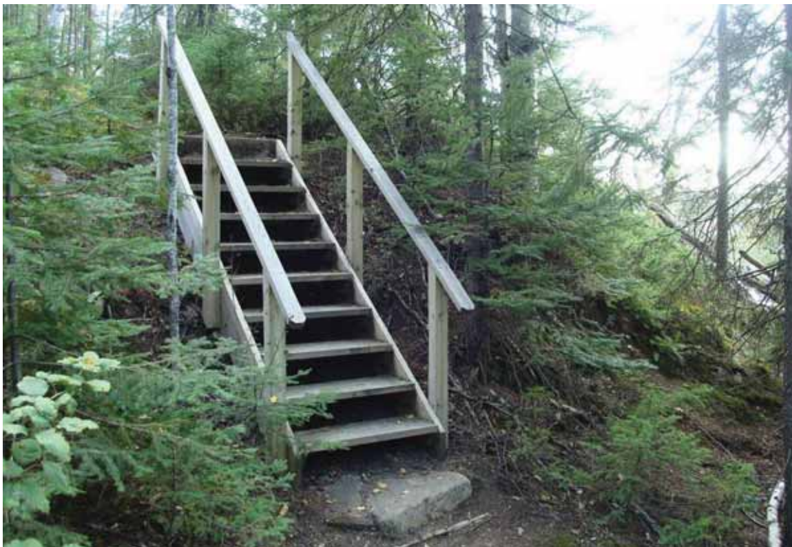
Figure 4- 42: Wood steps southwest of lodge, August 2012. (source: QEA)
