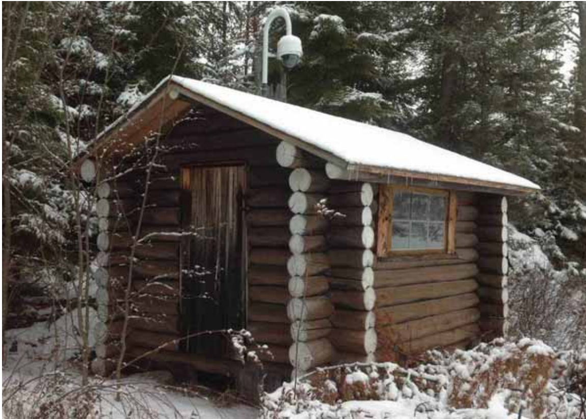
Figure 4- 31: Generator Shed, December 2012 (QEA)
