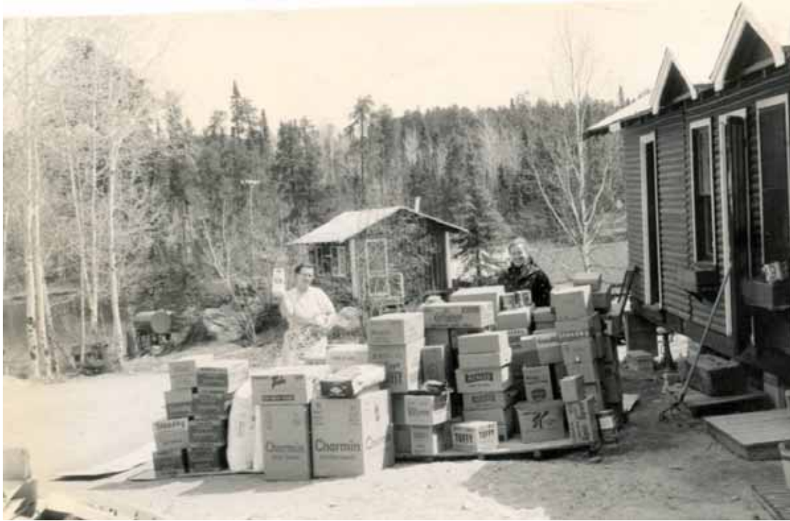
Figure 2- 25: Guest Cabin #1 (#4 Cabin), left and Laundry/Pantry/Dry Good Storage building, right, with spring supplies. (source: C-W 203)
