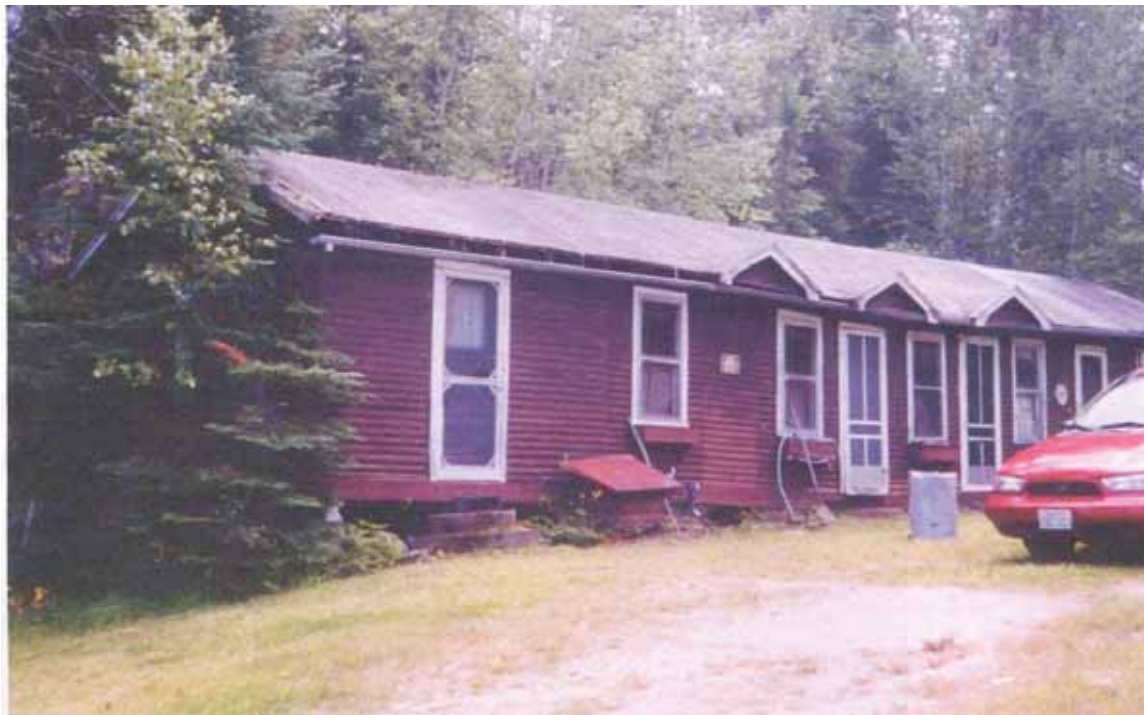
Figure 2- 11: Laundry/Pantry/Dry Good Storage building. (source: C-W 162)
