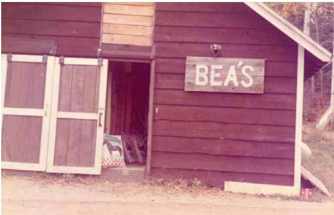
Figure 2- 40: Garage/ Ice House/ Fish Cleaning building, 1973. The sign was added for the Hamm's beer commercial. (source: C-W 181)
