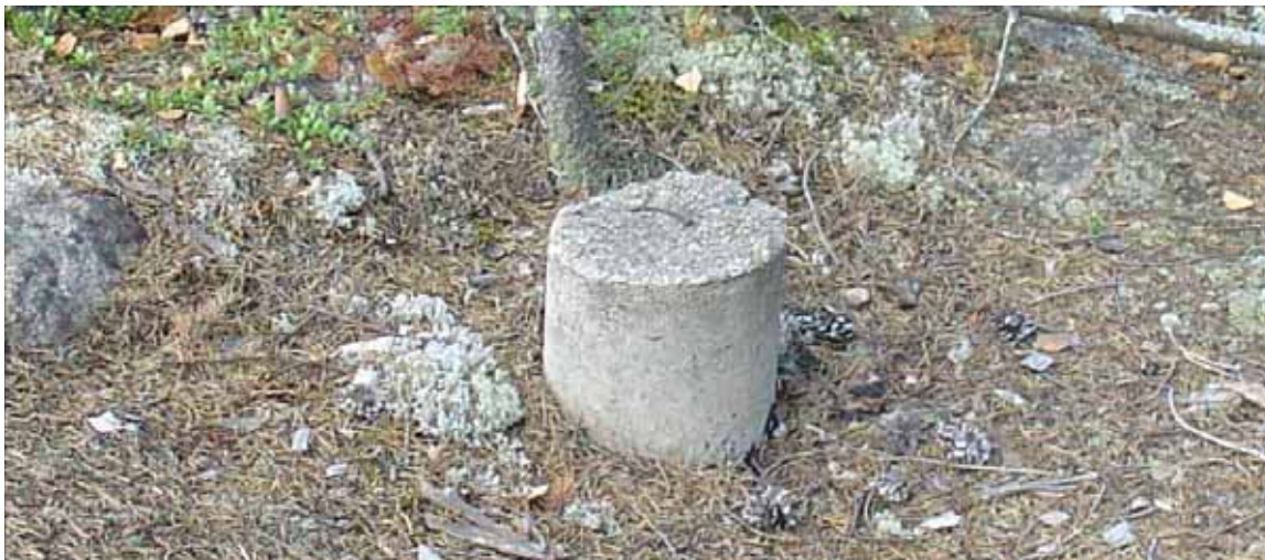
Figure 4- 34: Circular concrete cabin foundation post at cabin site, August 2012 (source: QEA)
