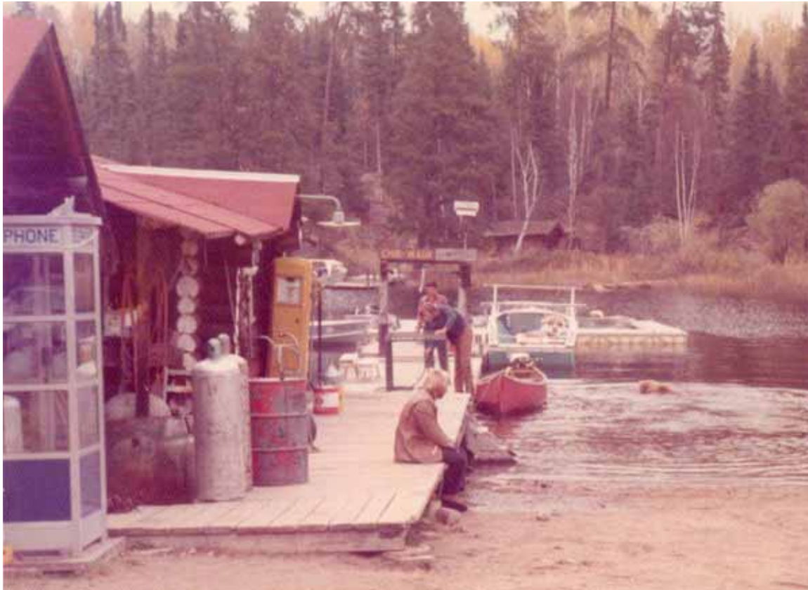
Figure 2- 31: Dock and adjacent buildings. Note building (#24) across the bay, 1973 (source: C-W 168)
