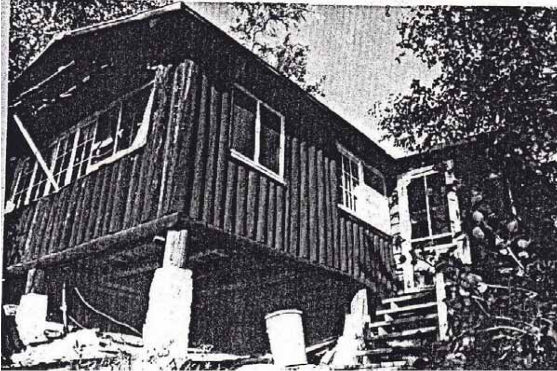
Figure 2- 62: Guest Cabin , #9 Cabin, date noted is ca. 1936 but more likely to be 1980. (source: USFS)
